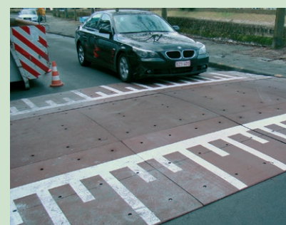
Extended Raised Table - Ghent in Belgium
