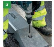
» Using an SDS drill with the 14mm drill bit provided, carefully and vertically drill out the holes to a depth of 110mm. Tip: Mark depth on bit using tape 240mm up from the drill point.
