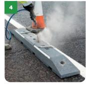
» Blow out the holes using compressed air to clear out any residue/dust left from the drilling. Note: Wear eye protection.
