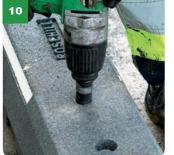
» The screws should then be hand turned in and tapped gently to start. Crank down fully in a crisscross formation across the unit using a 19mm socket and air/electric impact driver (nut runner). Note: Using a manual hand ratchet will not provide sufficient torque and strength to tighten the screws sufficiently, and may affect the warranty due to poor installation.
