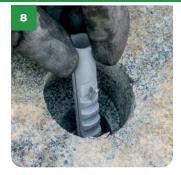
» Following on guickly behind, Insert the plugs into each hole.
