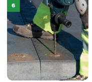
» Using an SDS drill with the 14mm drill bit provided, carefully and vertically drill out the holes to a depth of 110mm. Tip: Mark depth on bit using tape 240mm up from the drill point.
