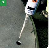
» Clip the anchor resin cartridge to the cage gun, cut off the end, attach the nozzle and squeeze the trigger to pre-mix the two components in the nozzle until a uniform mix exudes. Use the spent Roadfix container.
