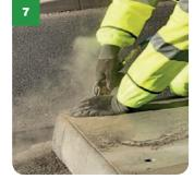
» Blow out the holes using compressed air to clear out any Roadfix residue/dust left from the drilling. Note: Wear eve protection as Roadfix adhesive can be forced up the holes with the dust.
