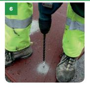
» Using an SDS drill and the 14mm drill bit provided, carefully and vertically drill out the holes to a depth of 110mm. Tip: Mark depth on bit using tape.
