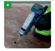
» Clip the anchor resin cartridge to the cage gun, cut off the end, attach the nozzle and squeeze the trigger to pre-mix the two components in the nozzle until a uniform mix exudes. Use the spent Roadfix container.
