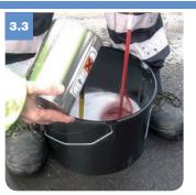
» Using a second person, slowly add the liquid from the metal tin (part A), pouring over 20 seconds whilst continuing to mix.
