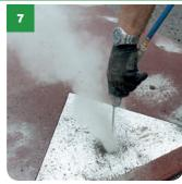
» Blow out the holes using compressed air to clear out any Roadfix residue/dust left from the drilling. Note: Wear eye protection as Roadfix adhesive can be forced up the holes with the dust.
