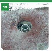
» Following on quickly behind, Insert the plugs into each hole and tap down until they are through and past the metal base bracket. Note: Forcing the coach screw and plug through together will only expand and damage it, preventing full penetration.
