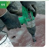
» The screws should then be hand turned in and tapped gently to start. Crank down fully in a crisscross formation across the cushion using a 19mm socket and air/electric impact driver (nut runner). Note: Using a manual hand ratchet will not provide sufficient torque and strength to tighten the screws sufficiently, and may affect the warranty due to poor installation.
