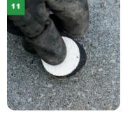
» Apply a small amount of the remaining anchor resin to the bolt heads of the shallow holes (thin covers) and the side wall of the thicker covers for the deeper holes. Fit the screw covers using a flat screwdriver to guide in.
