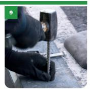
» Tap the plugs down until they are through and past the metal base bracket. Note: Forcing the coach screw and plug through together will only expand and damage it, preventing full penetration.
