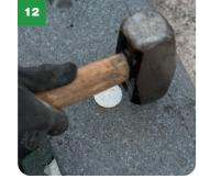
» Tap in flush with a lump hammer » Dispose of all fixing waste and wipe off any residue.
